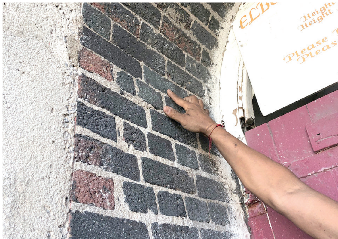
► The Elbow Reef lighthouse's uncovered brick.
