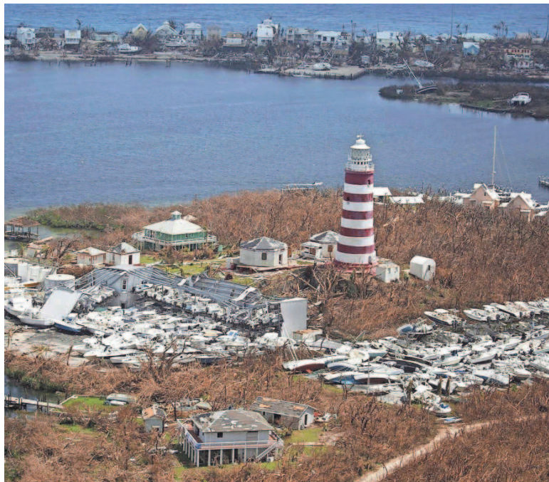
An aerial view of the Hope Town Lighthouse taken three days after Hurricane Dorian made landfall in the Abaco Islands of the Bahamas. NORTHWEST FLORIDA DAILY NEWS
